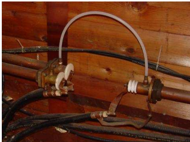
Figure 14.52: Flexible coaxial cables connected to rigid lines.
